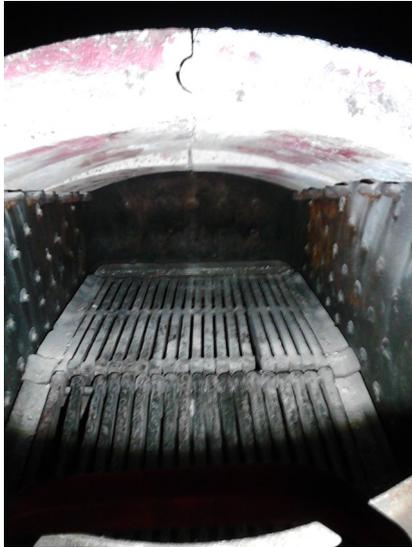
The last fire brick has been fitted into place – it caused more trouble than all of the others combined, as it had to be removed and trimmed three times before it slotted into place properly. Geoff was quite pleased to see it finally in place!
