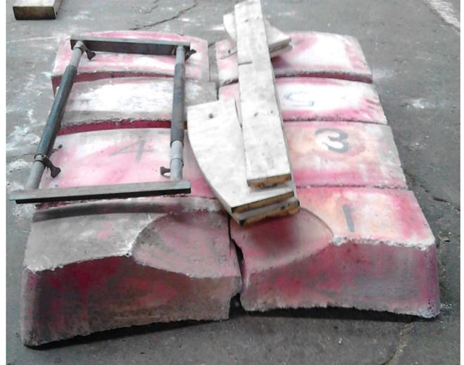
*The old fire bricks which form the brick arch that have been removed, shown with the installation tools to install the new fire bricks.*
