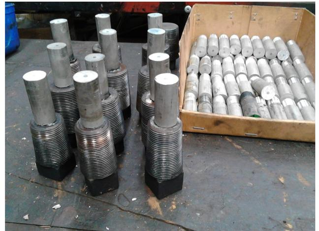
*The boiler plugs fitted with new anodes.*
