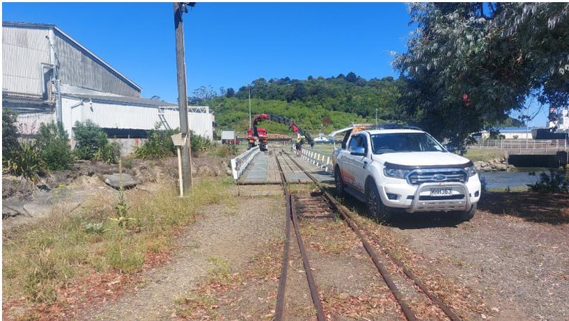
*Figure 1: C.R.Taylor fitting a replacement support post*
