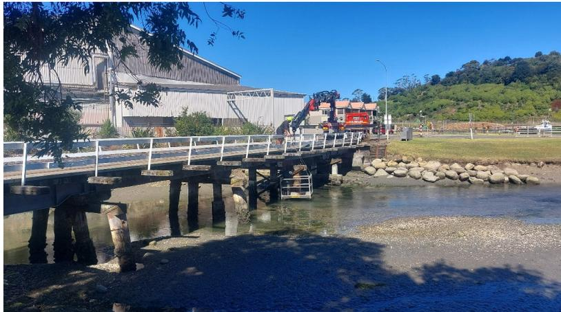
*Figure 2: C.R.Taylor fitting a replacement support post*
